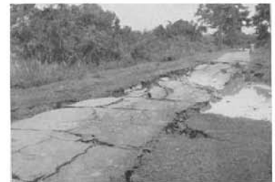
Cracks and subsistence in Upper Assam Trunk Road, Khowang
