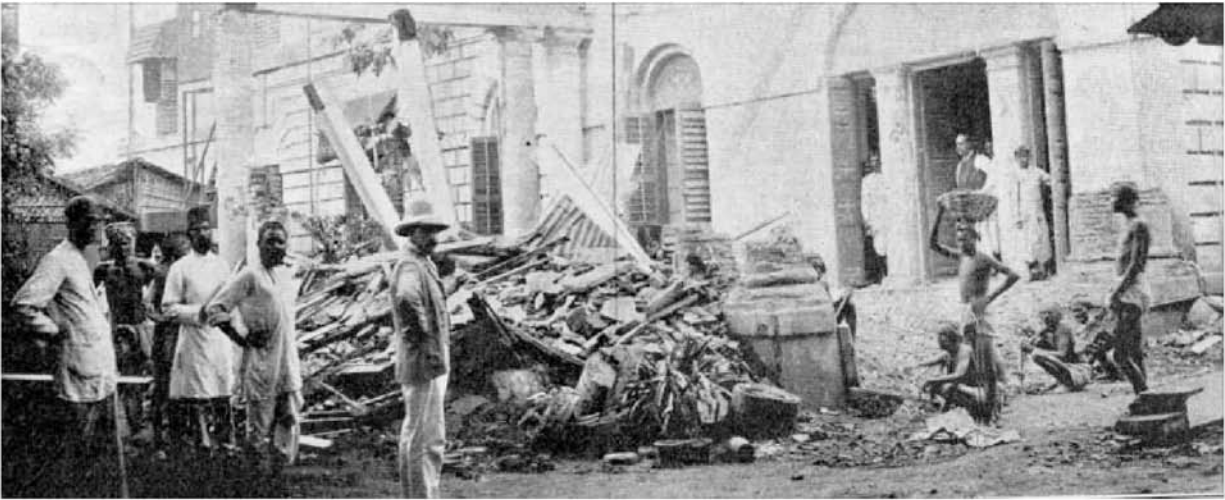
A collapsed portico in Calcutta due to Shillong Earthquake of 1897. The picture appeared in an article written by LaTouche ten days after the earthquake, and published 22 July 1897. In his article LaTouche emphasizes shoddy construction as the chief reason for building collapse in the city.
