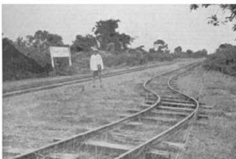
Loop formed on railway lines at Dangari
