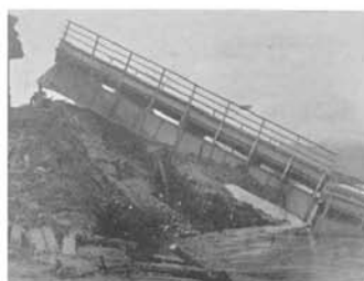
Bridge on Ranganadi North Lakhimpur
