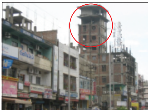
Beams are not spaced in regular geometry
