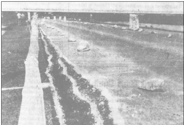
Figure 2 : (b) Damage of the National Highway in the Nowgong area caused by the Manipur-Burma border earthquake of August 6, 1988.
