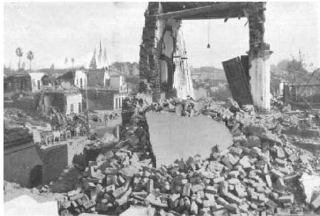
Damaged building in Guwahati after 1950 earthquake
