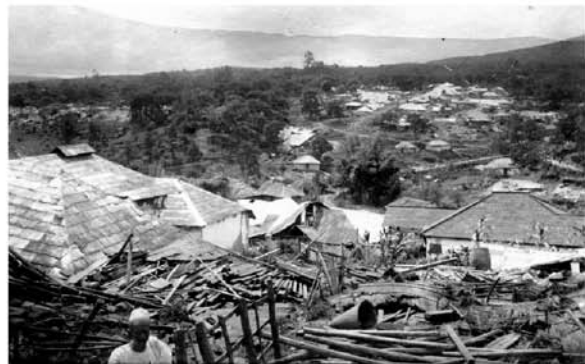
Flattened buildings, Shillong after 1897 earthquake.
