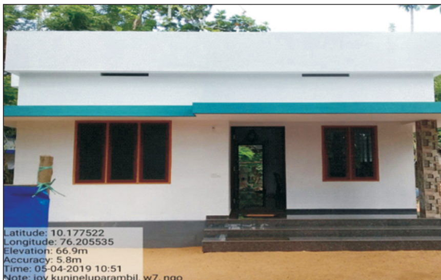
Figure 8.1 : Completely damaged houses rebuilt after the Kerala Floods, 2018
