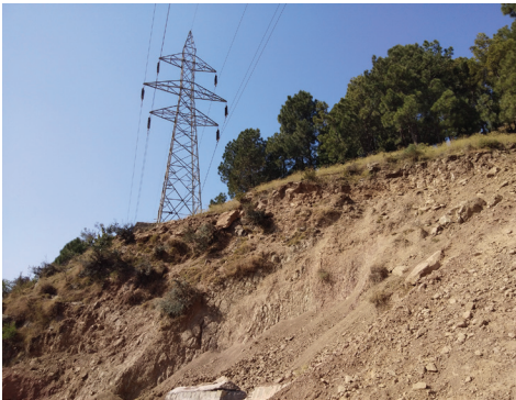
Photo 15: High Tension Tower Ch 87 + 505 km
