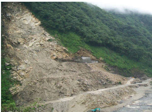
Fig. 5.5: Site condition before the start of work
