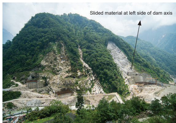
Fig. 5.4: Protection works for unstable portion
