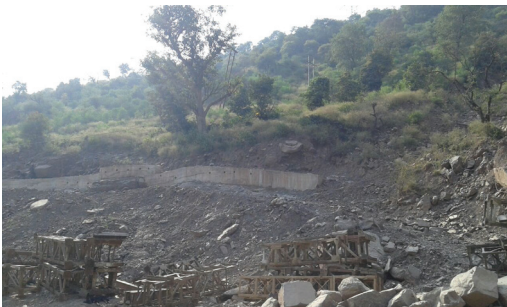
Photo 9: Geological strata at Ch 81 km, Narsoo village
