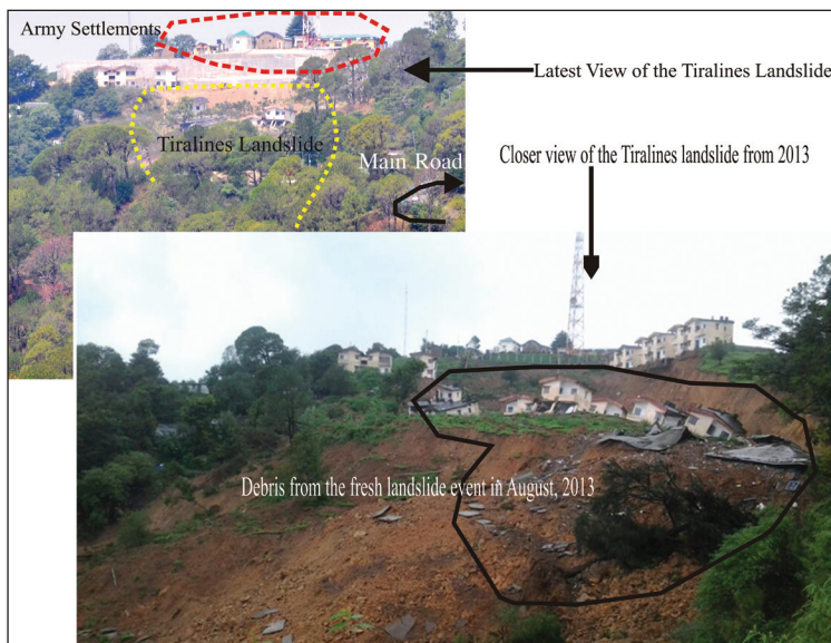
Fig. 11.2: View of the Tiralines landslide from August 2013 showing amount of damage and the latest view of the area showing the settlements just above the damaged slope
