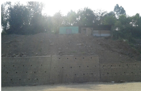
Photo 10: Geological strata at Ch 82 km, Narsoo Village
