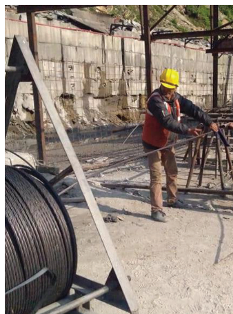
Fig. 5.6: Before commencement of cable anchoring
