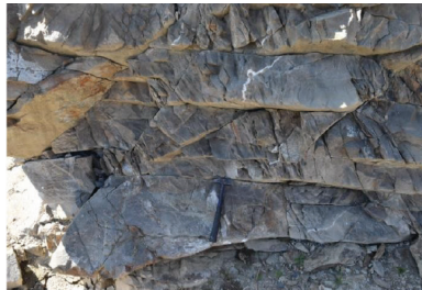
Fig. 3: Fractures and joints
