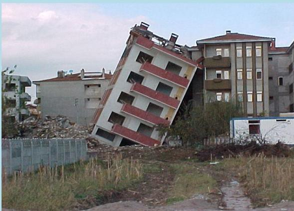
**Liquefaction induced bearing capacity failure during an earthquake (1999) in Adapazari, Turkey**
