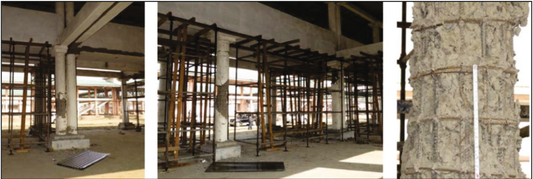
Figure 46: - Retrofitting of RC column by replacing circular ties with helical reinforcement
