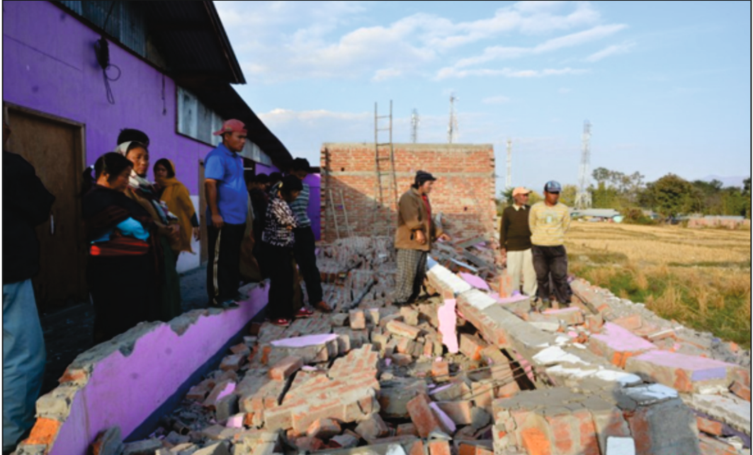
Figure 34: - Collapsed masonry building at Leimakhong area Manipur.
