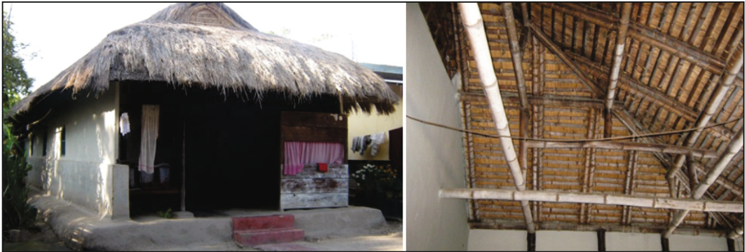
Figure 9: - Exterior look and roofing pattern of a typical Yumjao house
