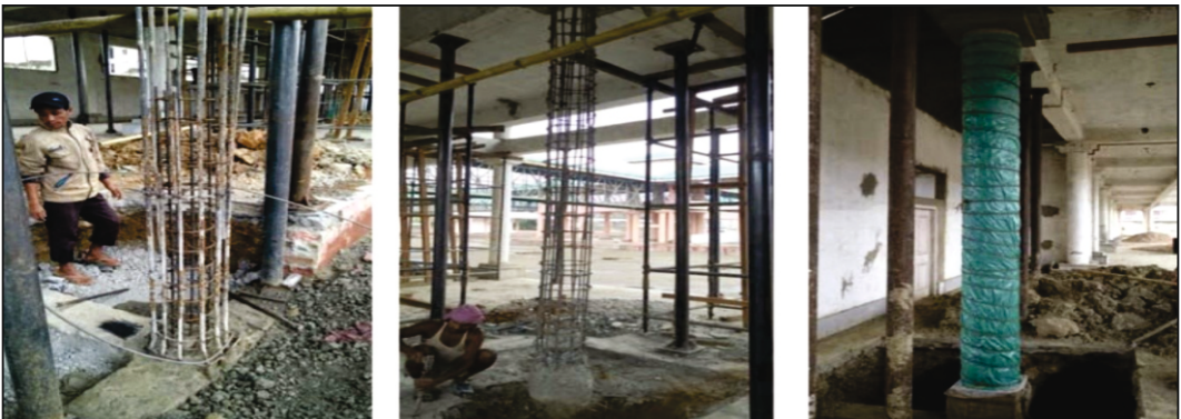
Figure 46: - Retrofitting of RC column by replacing circular ties with helical reinforcement
