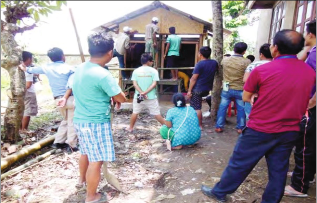
Figure 43: - Bamboo based Toilet Building at Imphal, Manipur.
