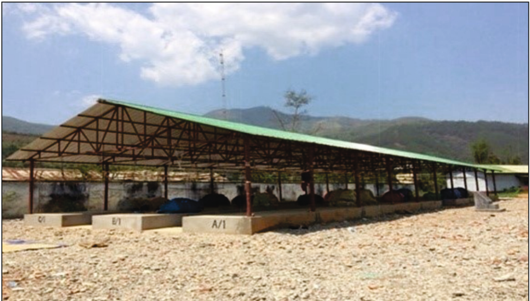
Figure 41: - Interim market space for women vendors built after the earthquake in Saikul
