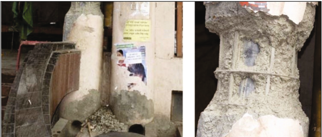
Figure 31: - Concealed drain water pipes inside the exterior columns
