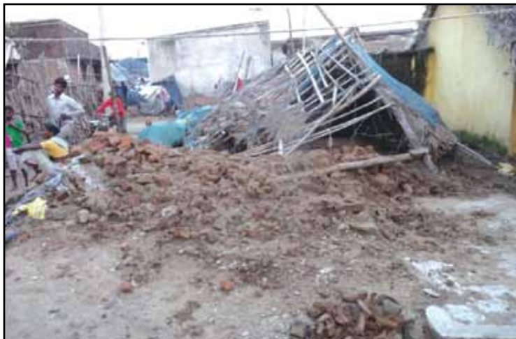
Figure 8: Damaged houses in Odisha
