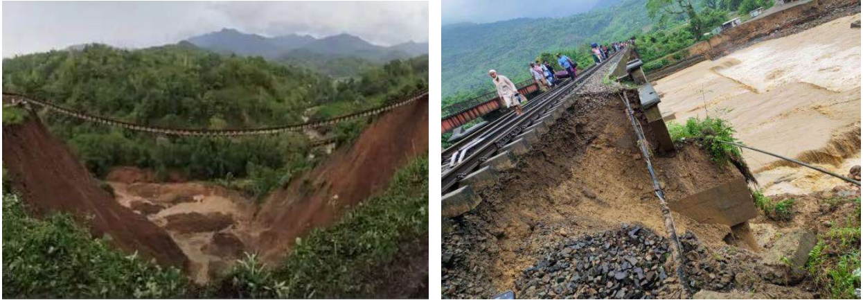
Figure 6: Railway track affected by rainfall-induced landslide along on 14 May 2022. (Roy et al., 2022; The Federal, 2022)
