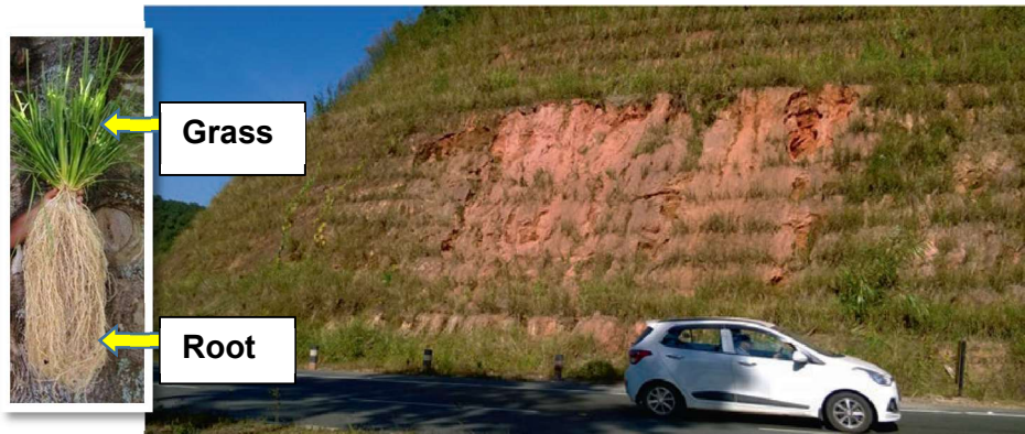
Use of Vetiver grass in the cut-slope – affordable and naturally stabilised
