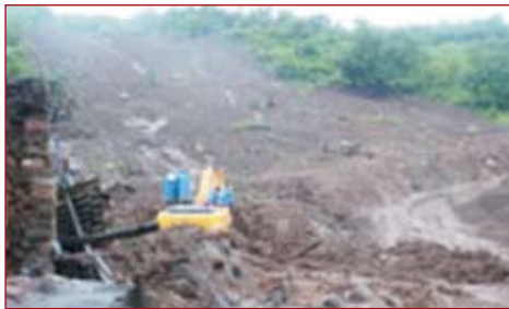
Rescue work during the landslide
