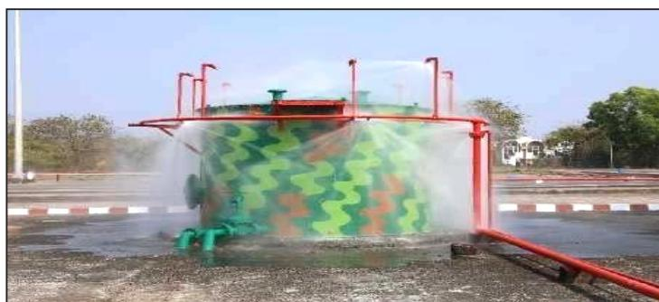
Figure 62 Fixed Water Spray System
