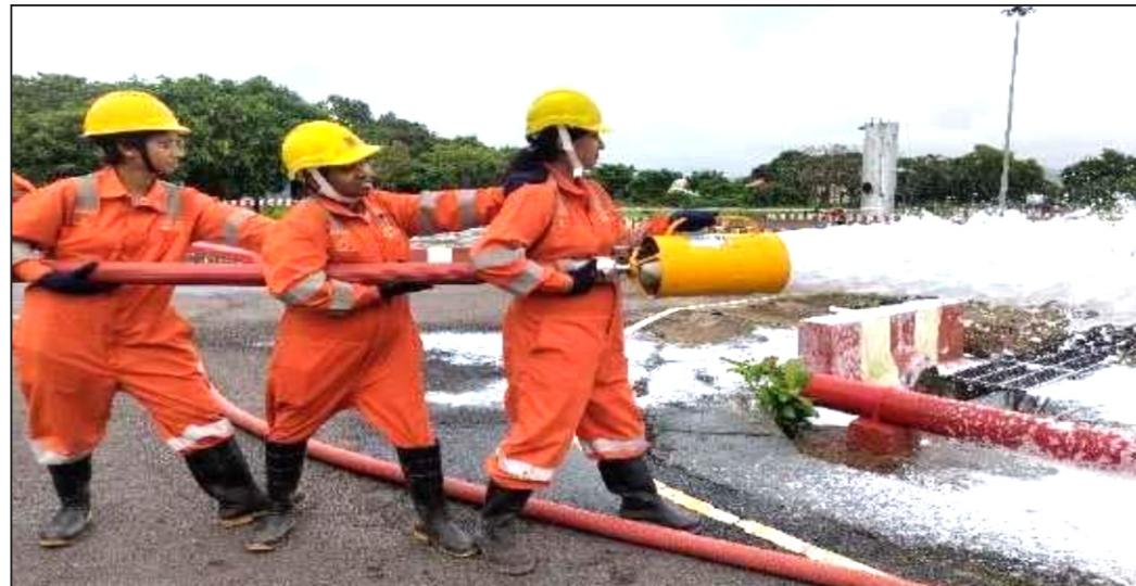
Figure 48 Foam being discharged through MEGF
