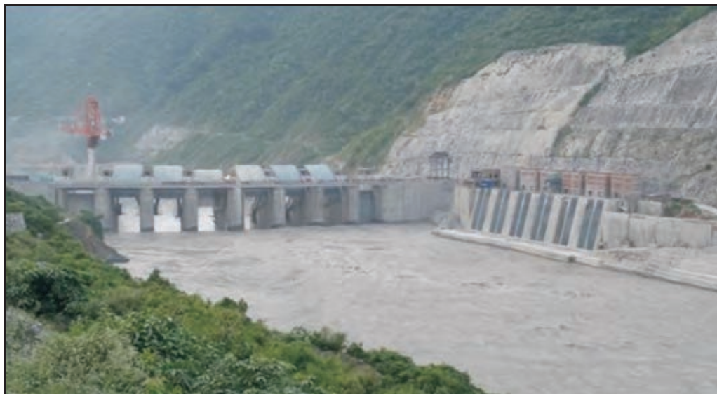
Figure 2.8: Hydel power project in Srinagar, Uttarakhand 44 .
