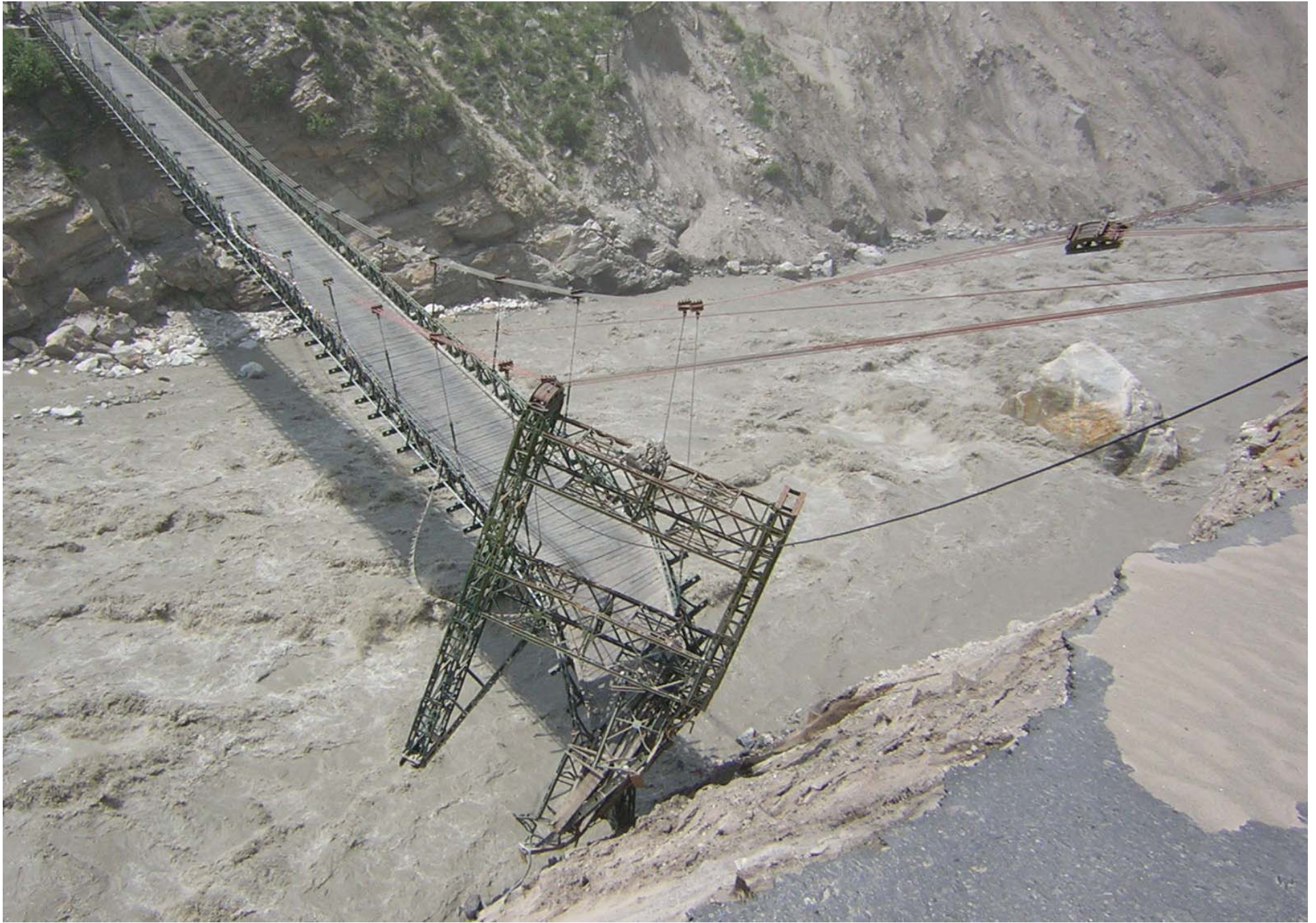
360 FT BSB AKPA BRIDGE HANGING ON ROPE
