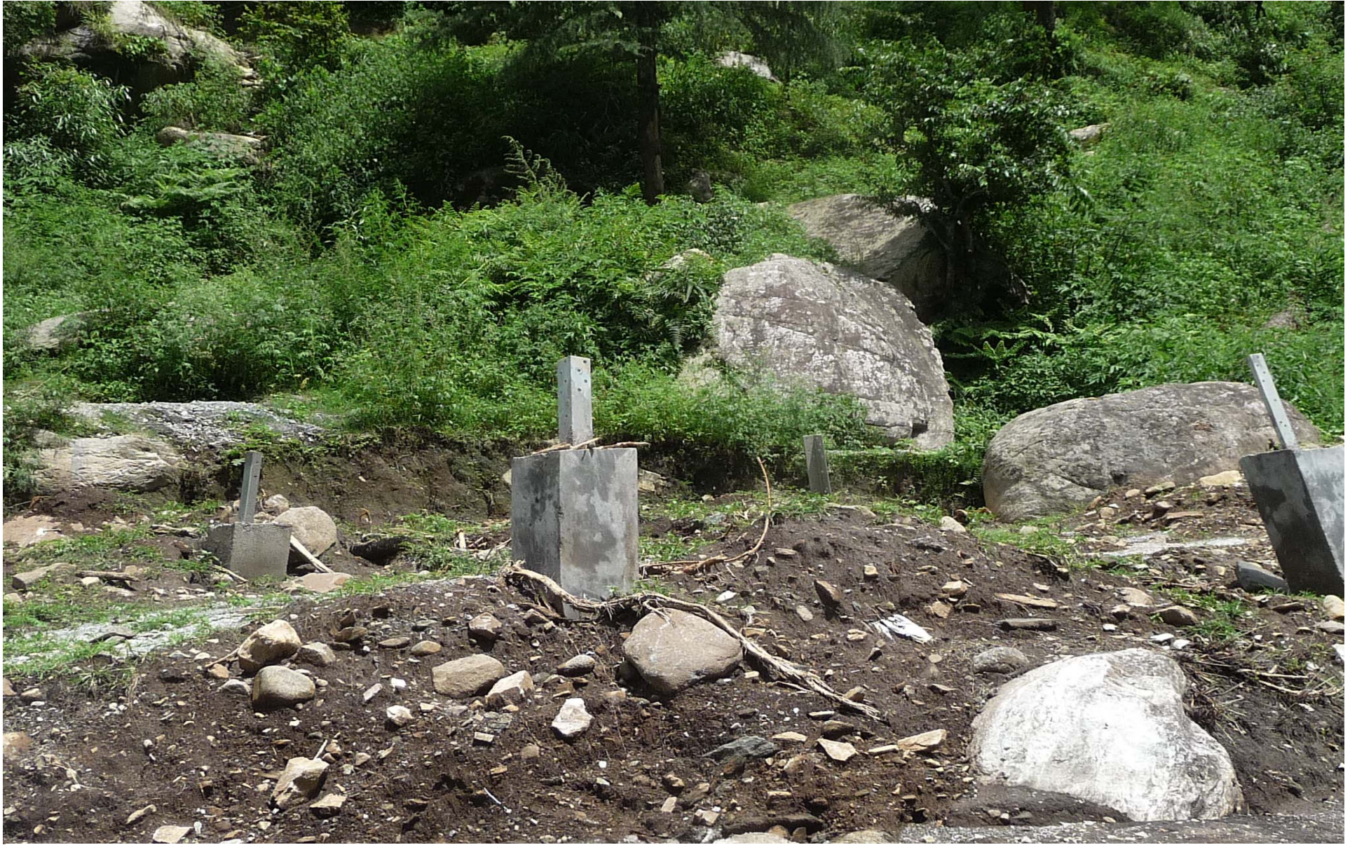
Fig.11: Transmission Tower location affected adversely after the flashfloods in Asi Ganga Valley
