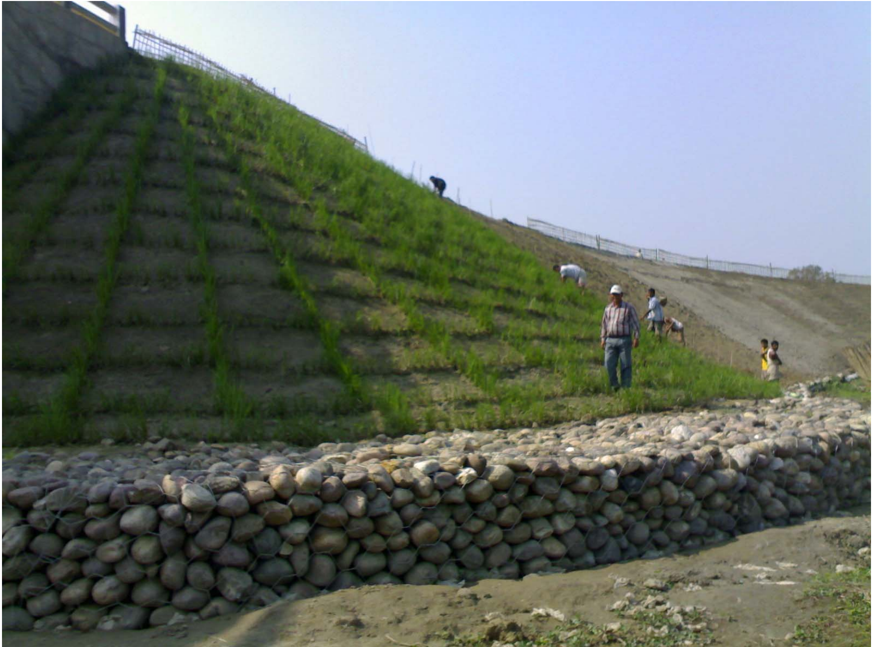
Slope protection with vetiver and forward slope toe protected with caged boulder
