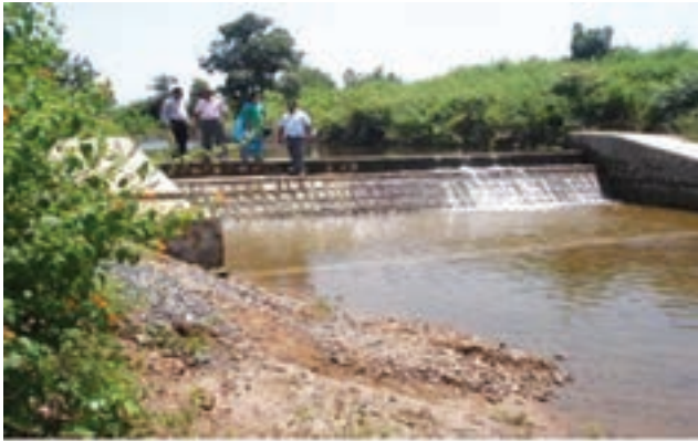
Figure 3.5: Structural Mitigation Measure (Stop dams) in Chopra Village, Datia
