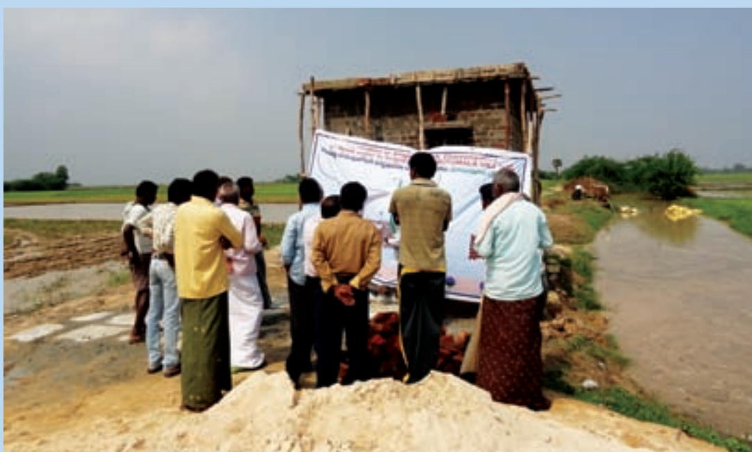
Pic 4: Renovation of irrigation tank, channelization of flood water to irrigation tank, Motumala, AP
