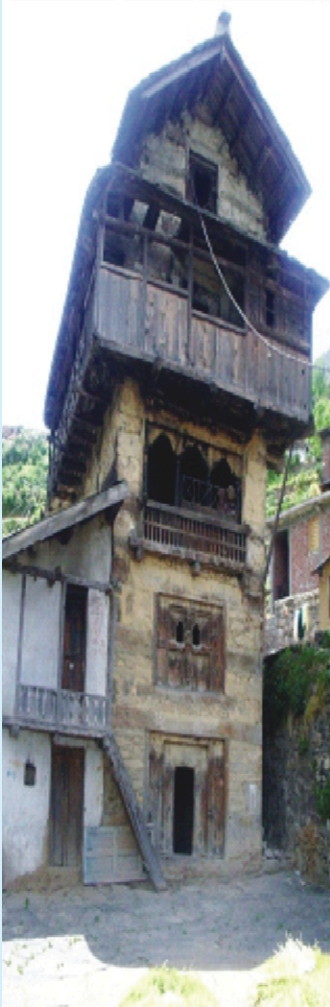
350 Year Old Building at Uttarkashi
