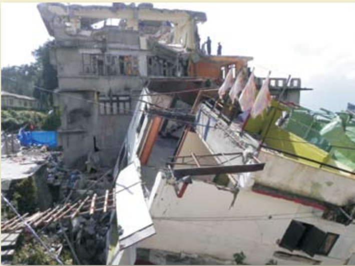
Two buildings at Baluakhani developed excessive tilt on 23rd Sept 2011. Special team from Hyderabad was engaged for demolition. Several buildings in Gangtok have been declared unfit and they are being demolished one by one. However, there is a need to look into the safety of these buildings by experts.
