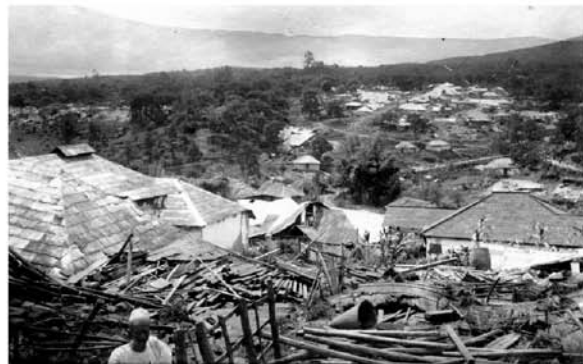
Flattened buildings, Shillong after 1897 earthquake.
