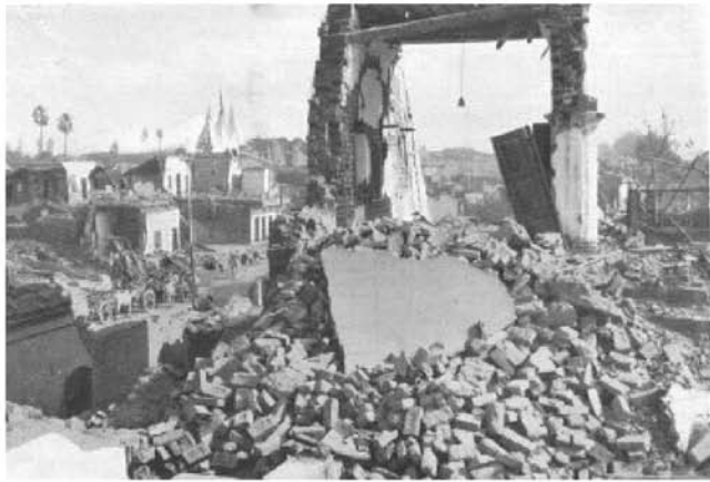
Damaged building in Guwahati after 1950 earthquake
