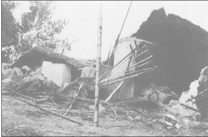
Figure 2 : (a) Damage of a mud hut in the Cachar area caused by the earthquake of December 30, 1984.
