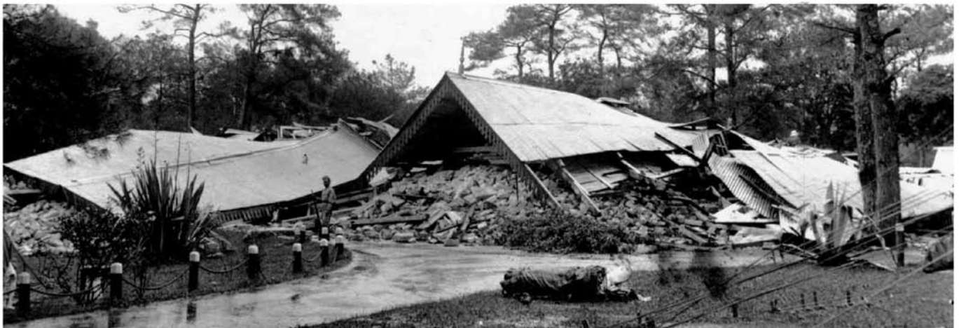
Ruins of Government House Shillong after the earthquake
