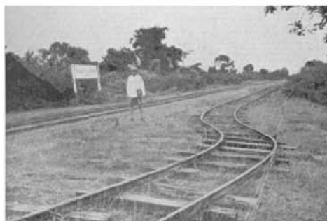
Loop formed on railway lines at Dangari
