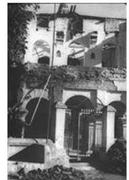
Temple at Dibrugarh damaged by the earthquake of 1950
