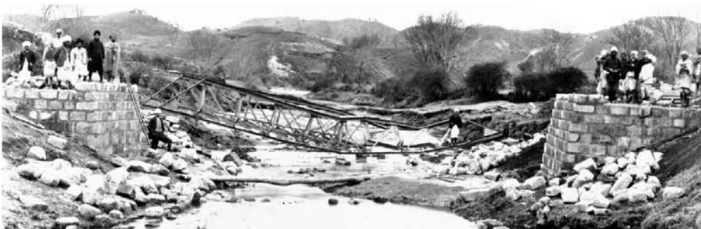
Collapsed bridge outside of Shillong thrown from its abutments by the earthquake. Mrs. Sweet and Mr Monaghan had just ridden across it. In his official report LaTouche states: "The large bridge on the Gauhati road about 1.5 miles from Shillong, over the Umkra River, has suffered severely. The abutment on the SE side fell entirely carrying the girders with it. The two piers and the abutment on the northwest side which are of more recent construction, remained standing though somewhat cracked."
